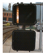
Vertical Bar Illuminated Proceed The light rail operator sounds the bell and proceeds through the intersection.
